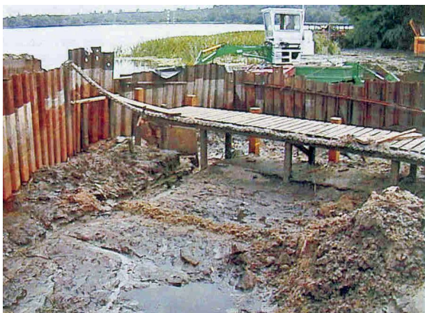
Dredging & Construction of Main Sailability Jetty 2001
