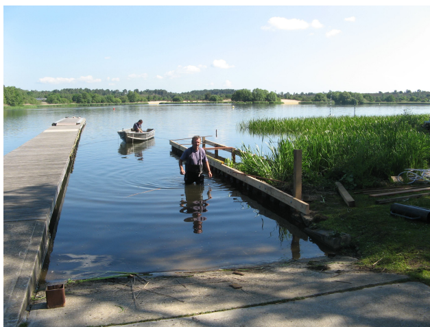
Construction of New Sailability Jetty 8 2007
