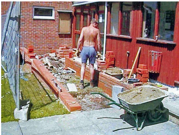
Construction of Clubhouse Access Ramp 2001
